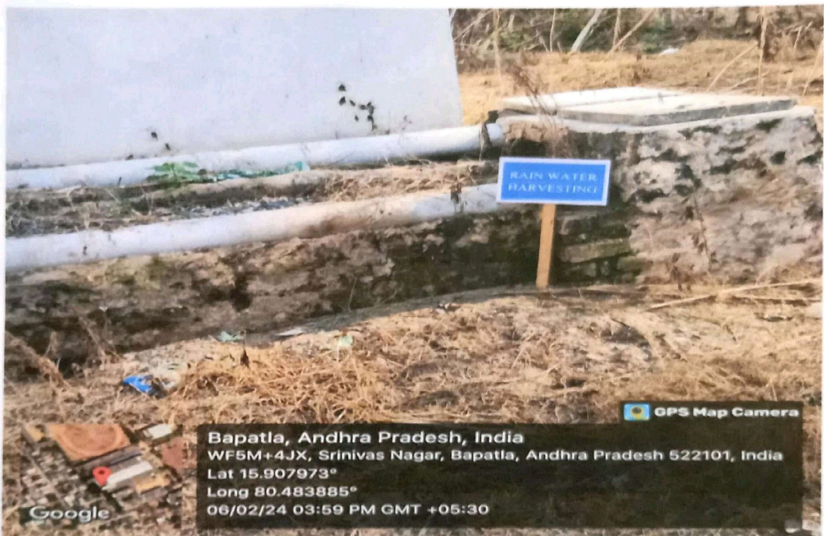
RAIN WATER HARVESTING
